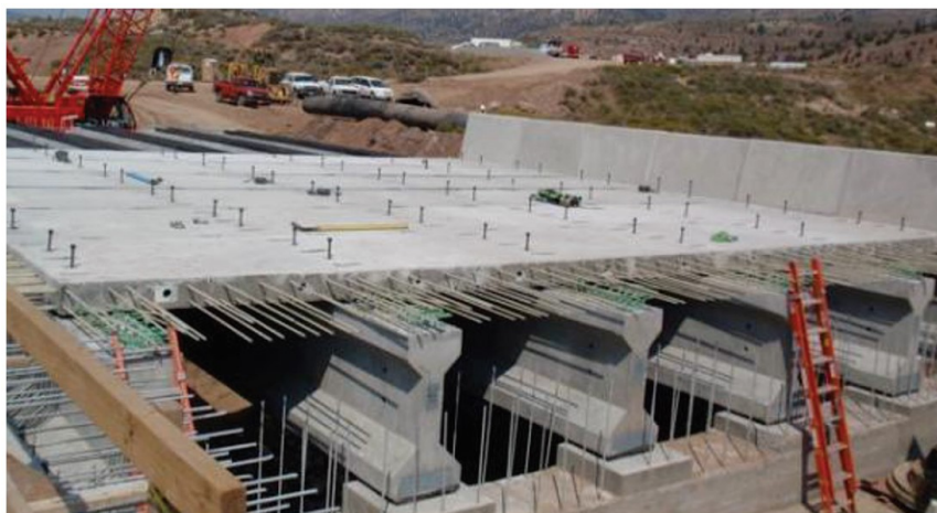
Figura 11 – Emma Park Bridge - Utah
