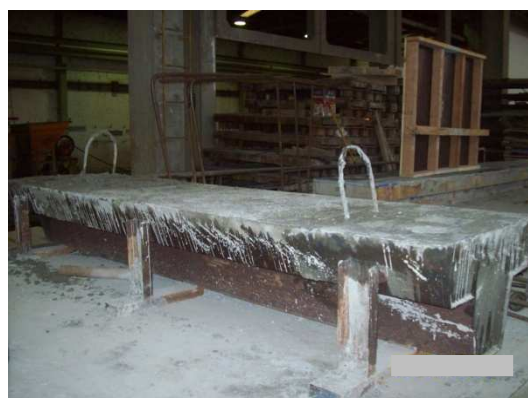
Figura 36: Viga com concreto fresco residual
